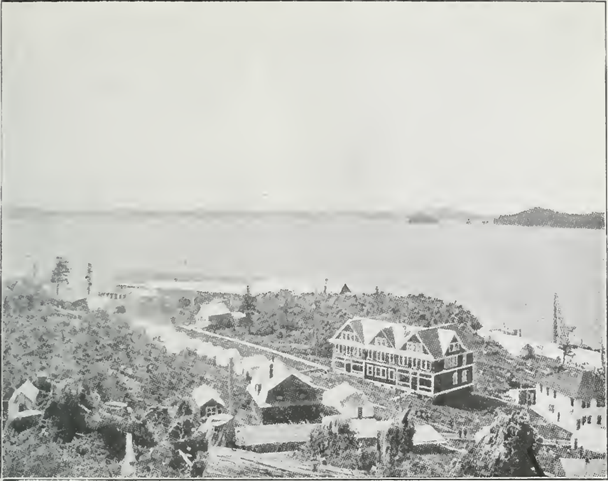
TEMPORARY RAILROAD HOTEL AT PRINCE RUPERT
